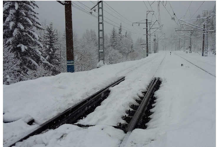
CLHS system in operation on Nanhchul station, Krasnoyarsk Railroad, Russia
